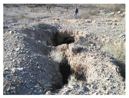
**Figure 2.2** Formation of jugholes in an auxiliary spillway of Diablo Arroyo Site 1, Hudspeth County, in the Trans-Pecos area of Chihuahua desert, USA (Image source: USDA NEH 633.13)
