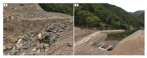
**Figure 4.1 a** Exposed section of the materials composing the Akatani landslide dam **b** Upstream side of the Akadani landslide dam showing water inflow into the dam through an artificial drainage pipe. Note: People for scale.
