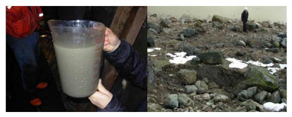
**Figure 7.17** Investigation of seepage in Howard Hanson Dam, USA. (**a**) Turbid water collected from a vertical drain at the right abutment, (**b**) Occurrence of a large depression at the upstream slope of the right abutment.
