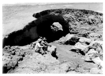
**Figure 1.15** The May 1937 piping failure of a dam in Arizona (USA) comprised of dispersive soil (Image source: USDA NEH 633.13)
