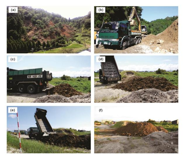
Figure 7.3 Early stages of construction of the dam models showing: (a) The landslide at Mihata district, near Izumo, Japan (b) Toe part of landslide from where the landslide materials were sourced ( $\mathbf{c} \sim \mathbf{f}$ ) Offloading of the landslide materials at the experimental site in Eshima Island.
