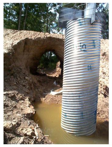
**Figure 2.1** The 2002 piping failure of the Lonesome Dove Reservoir levee in Louisiana, USA (Image source: USDA NEH 633.13)
