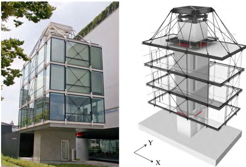
(a) Photograph (left) and perspective drawing (right) of first CSI-equipped building
