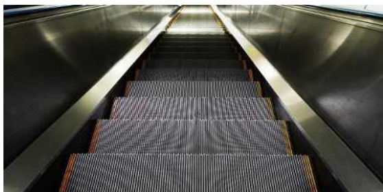
The bottom of the escalator
