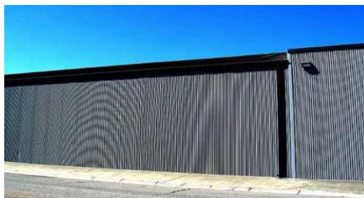
Appearance of building
