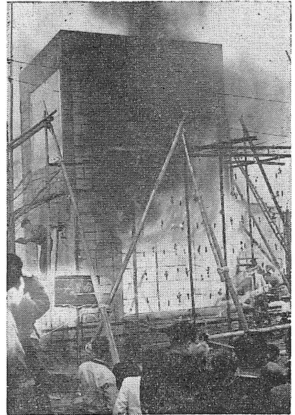
Fig. 6 A view of fire resistance test of leaves (1)
