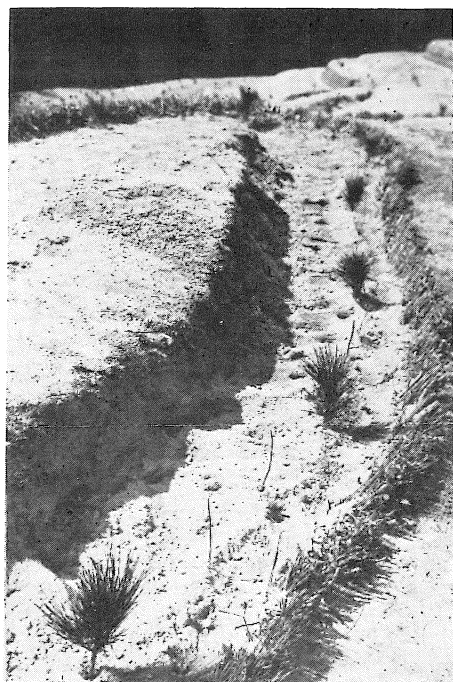
Photo. 2 Sujikô (terracing with fascine.)
