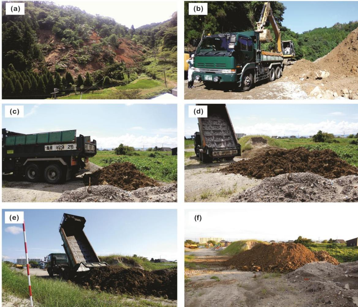
**Figure 7.3** Early stages of construction of the dam models showing: (a) The landslide at Mihata district, near Izumo, Japan (b) Toe part of landslide from where the landslide materials were sourced (c~f) Offloading of the landslide materials at the experimental site in Eshima Island.
