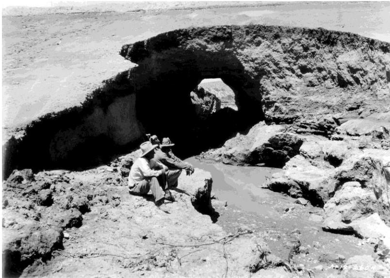
**Figure 1.15** The May 1937 piping failure of a dam in Arizona (USA) comprised of dispersive soil (Image source: USDA NEH 633.13)
