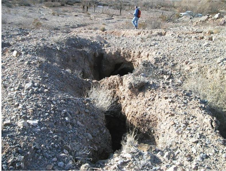
**Figure 2.2** Formation of jugholes in an auxiliary spillway of Diablo Arroyo Site 1, Hudspeth County, in the Trans-Pecos area of Chihuahua desert, USA (Image source: USDA NEH [633.13](#))
