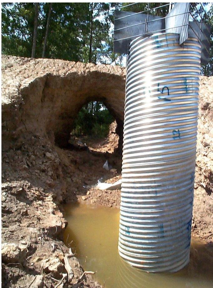
**Figure 2.1** The 2002 piping failure of the Lonesome Dove Reservoir levee in Louisiana, USA (Image source: USDA NEH [633.13](#))
