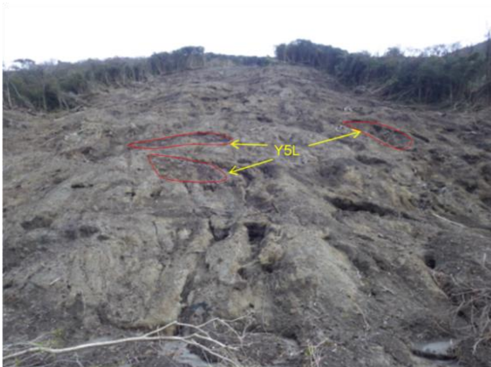
Fig. 5.11 Exposed slope after shallow landslide. Basalt (Y5L) is exposed in places.
