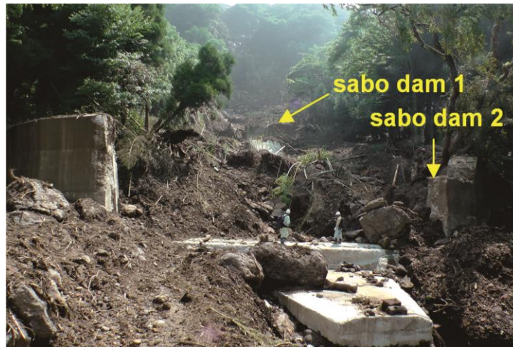
Fig. 4.12 Sabo dams destroyed by debris flow
