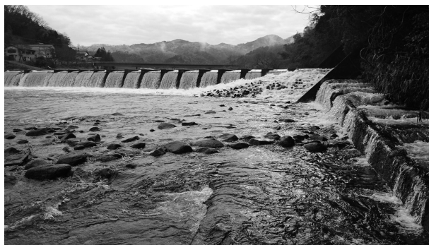
Figure 1 Yoshii fishway (taken from the downstream)
