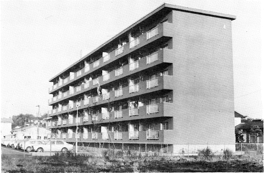
Photo. Apartment Building used for the Experiment (Length 56,200mm, Width 7,300mm, and Height 14,750mm)
